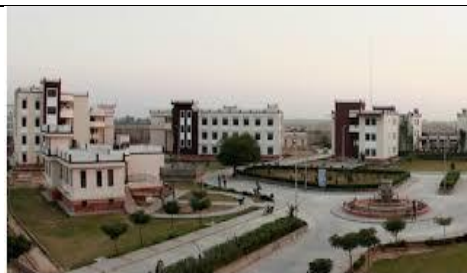
Jagannath University Village Rampura, Tehsil Chakshu, Jaipur (Rajasthan)
