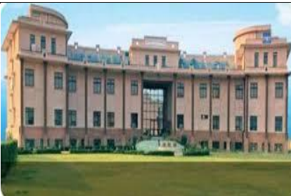
Jagannath Gupta Institute of Engg. & Technology Plot No. IP 2 & 3, Phase-IV, Sitapura Indl. Area, Jaipur (Rajasthan)
